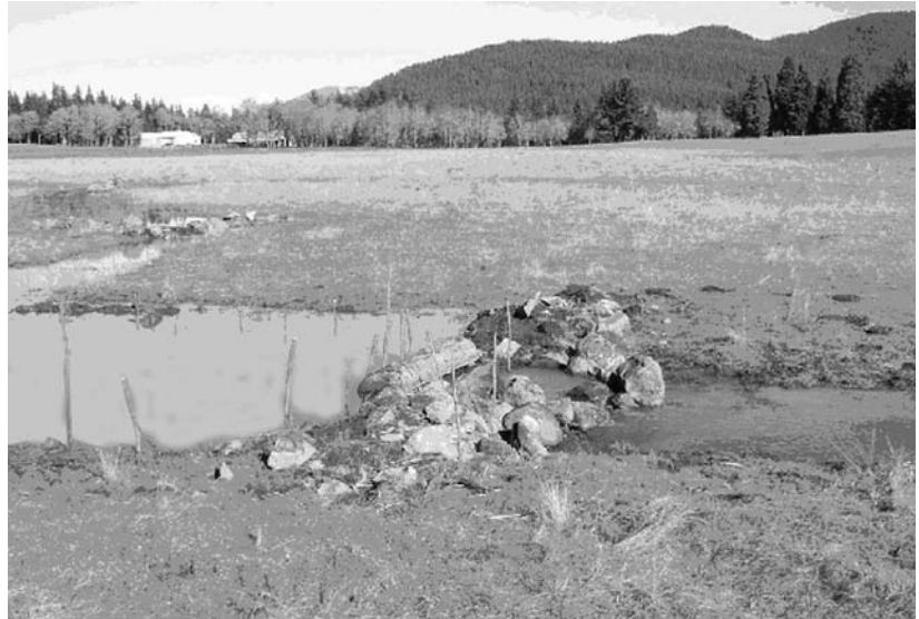
Figure 12. Blocked ditch with sticks. Old pasture drainage system blocked with low soil, rock, and wood dam and stabilized with live willow cutting stakes. Photograph taken after one winter rainy season. Photo by Rick Barney, NRCS
