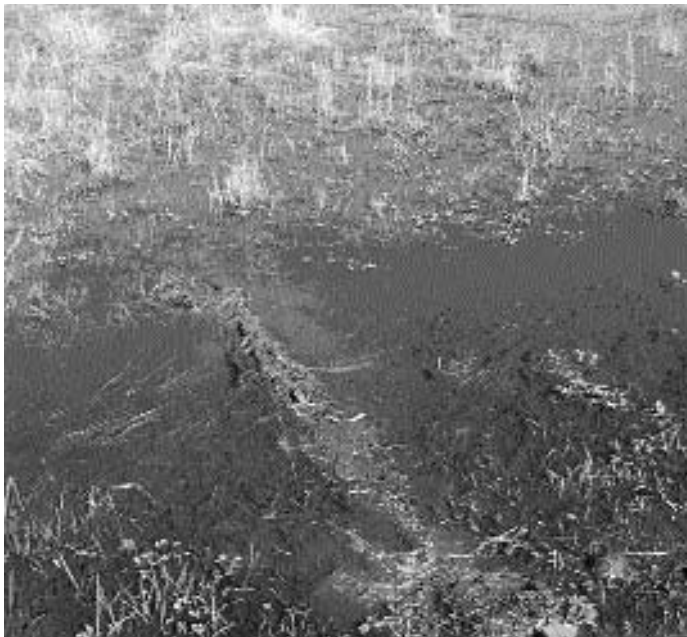
Figure 10. Bundle of cottonwood cuttings placed in a small ditch to slow run off and ultimately generate riparian vegetation through hardwood cutting. Photo by Rick Barney, NRCS
