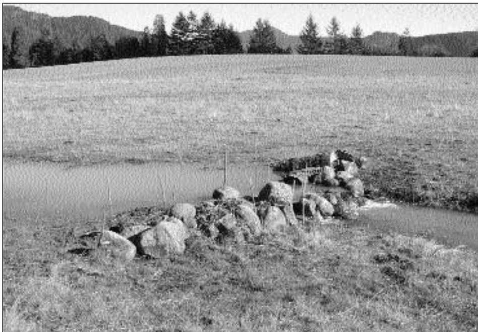
Figure 8. A low dirt berm reinforced with rock. Notice willow cuttings in place upstream of the berm. Photo by Rick Barney, NRCS.
